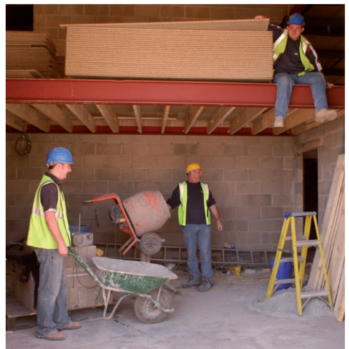
Broadreach House: Converting a factory building into a day support centre
